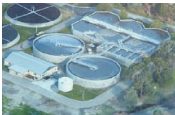
Figure 8.7 An aerial view of a sewage plant
